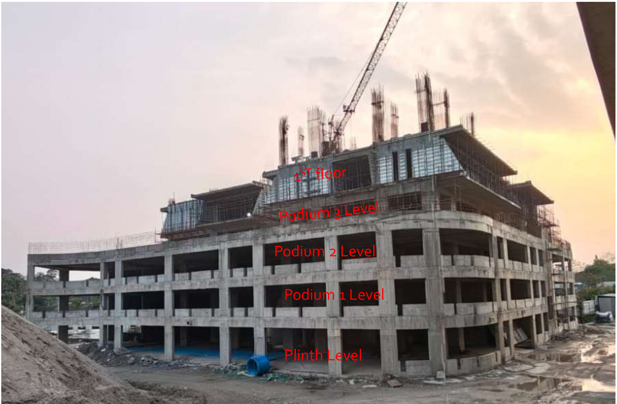
TOWER - B 1 ST TO 2 ND FLOOR SLAB CASTING COMPLETED.
